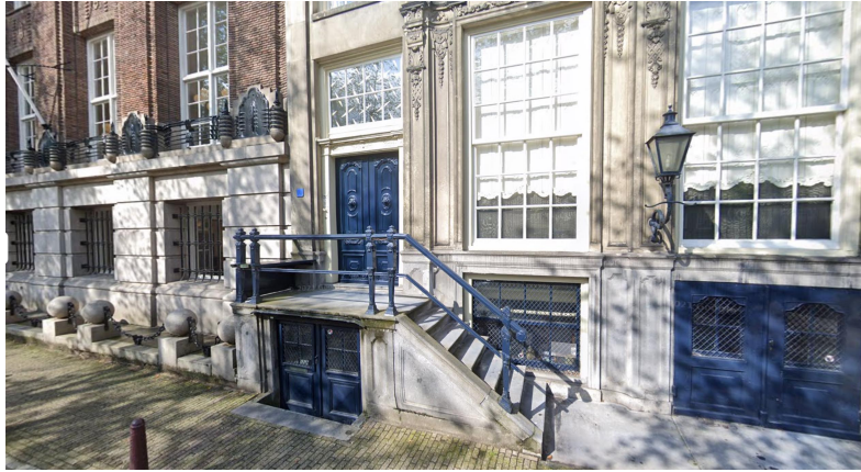
Figure 13: Example of a “half-floor” for a building in Amsterdam. Notice how the adjacent building does not have this half-floor. [Source: Google Street View (2022)]
